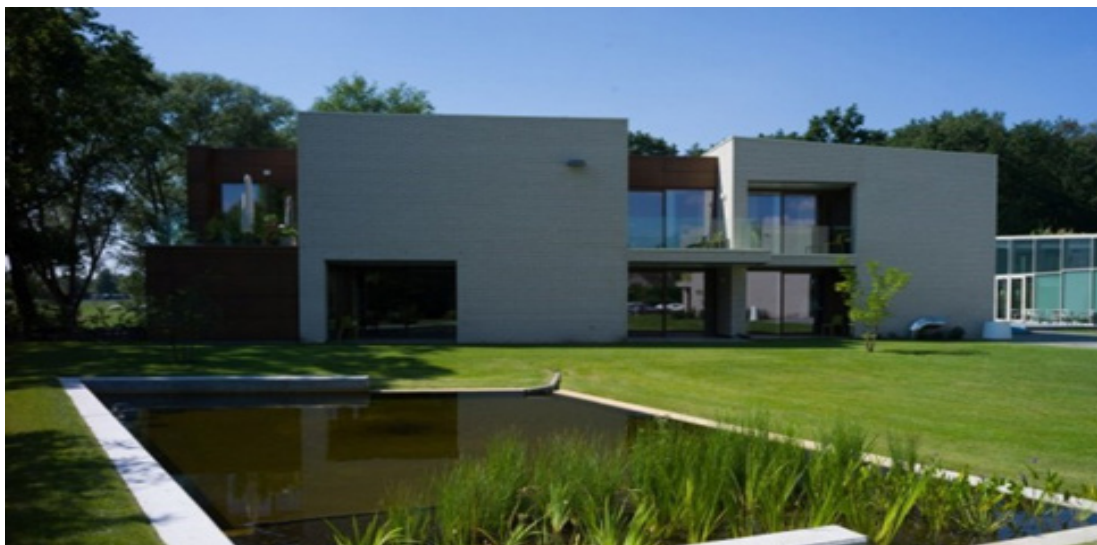
Group of assisted living apartments Ter Bleuk
